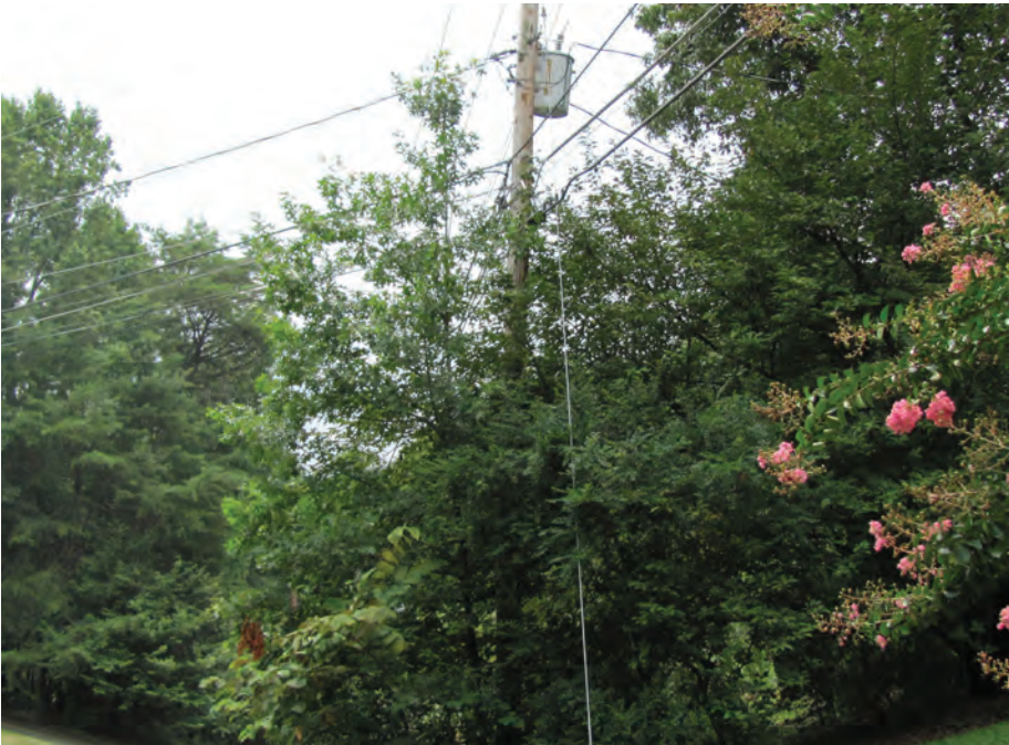
KUB clears unmaintained vegetation around poles for safe access.
