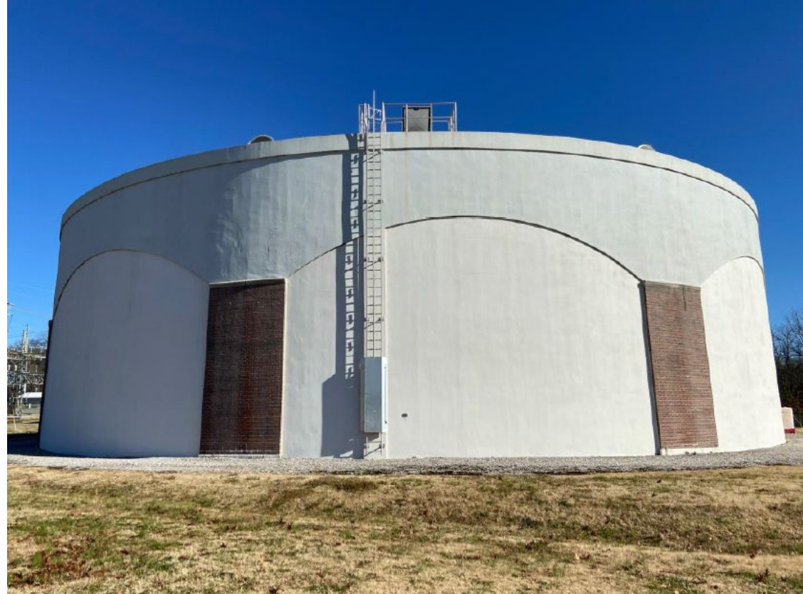
MBW West Clearwell
