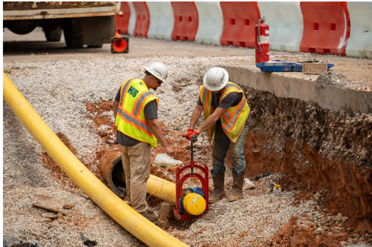
Gas Steel Pipe Replacement $5.0M
